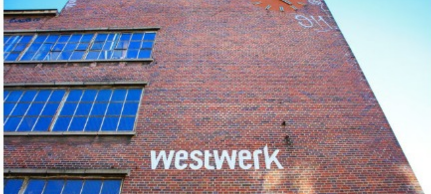
The Westwerk has post-industrial structures.
